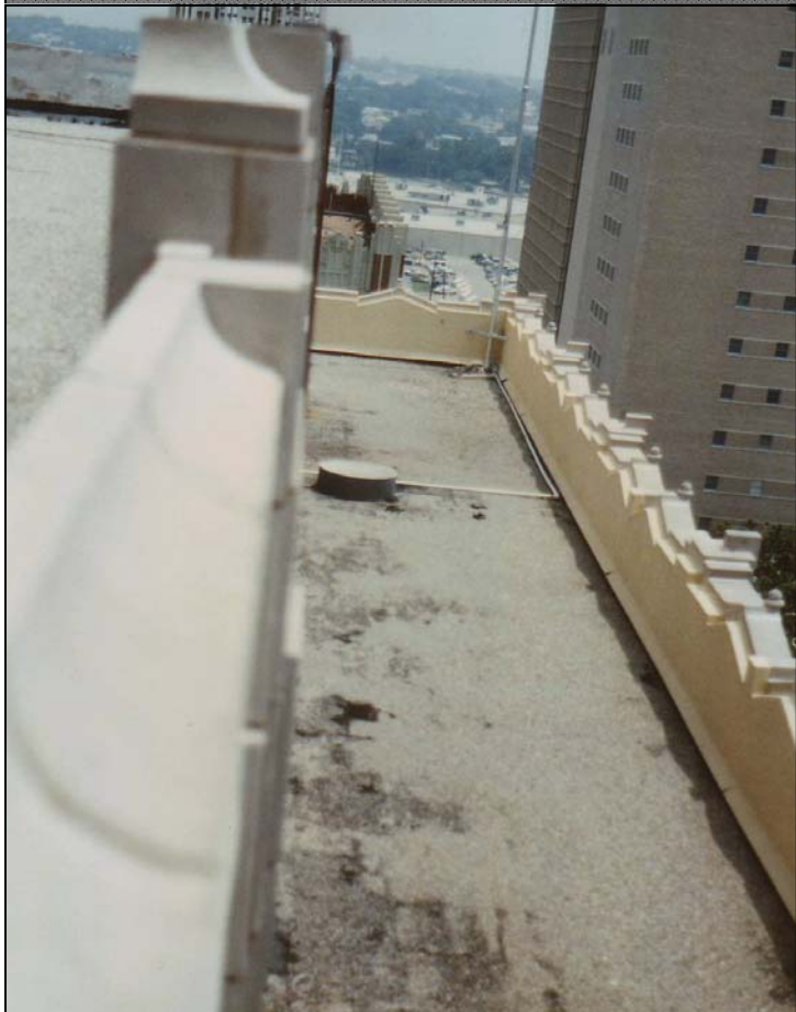
The Roof Garden from above facing NE (1989)
